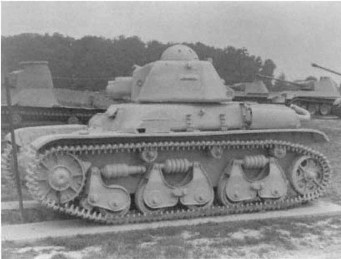
The Renault R-35 mounted a 35mm gun and was run by a twoman crew.
