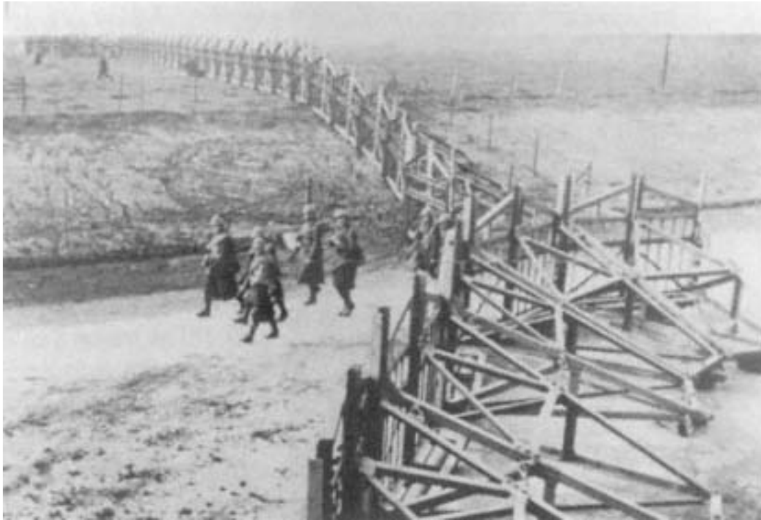
The Belgian Gates during the Phony War. This tank obstacle was an important part of the Belgian defensive line.
