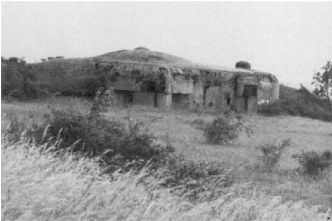
Block 3 at the small ouvrage of Rohrbach. View from the rear showing flanking embrasures for infantry weapons and a GFM cloche at the right. On the top is a machine gun turret in the eclipsed position.
