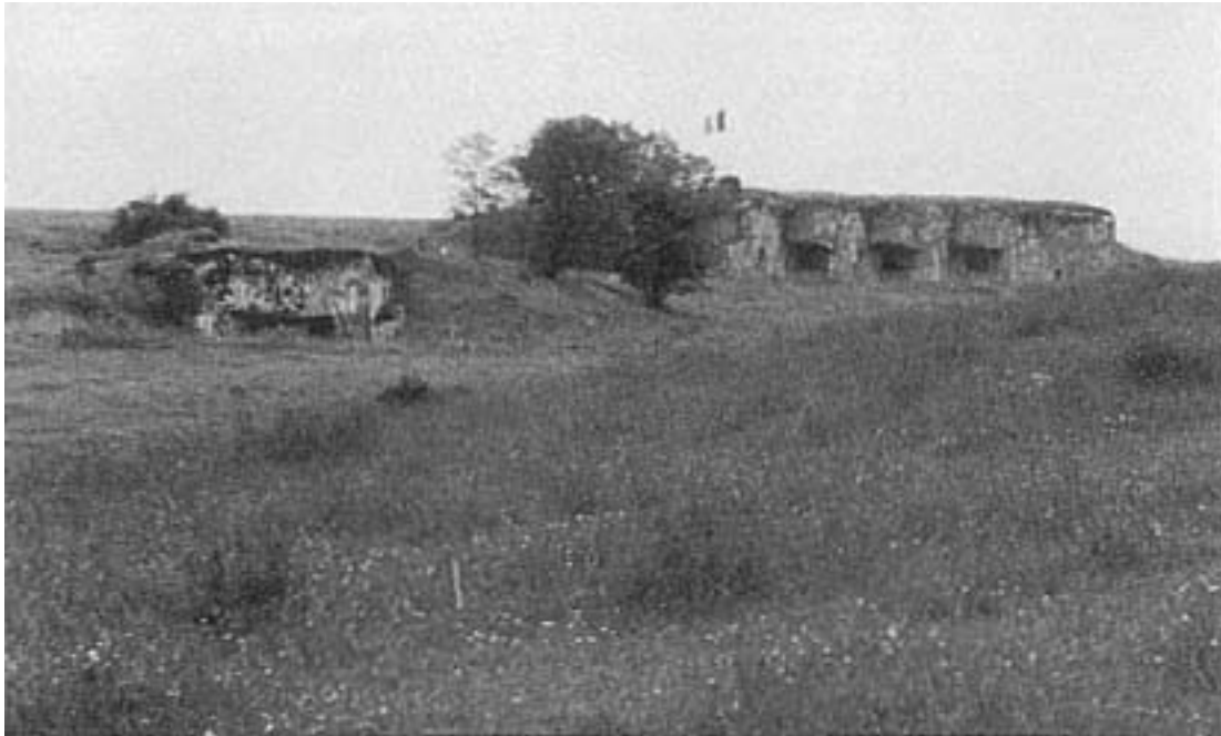
Artillery casemate (Block 4) and infantry casemate (Block 7) of Fermont. The three 75mm guns covered the right flank and infantry block on the right and with its 47mm anti-tank gun protected Block 4 from ground assault.
