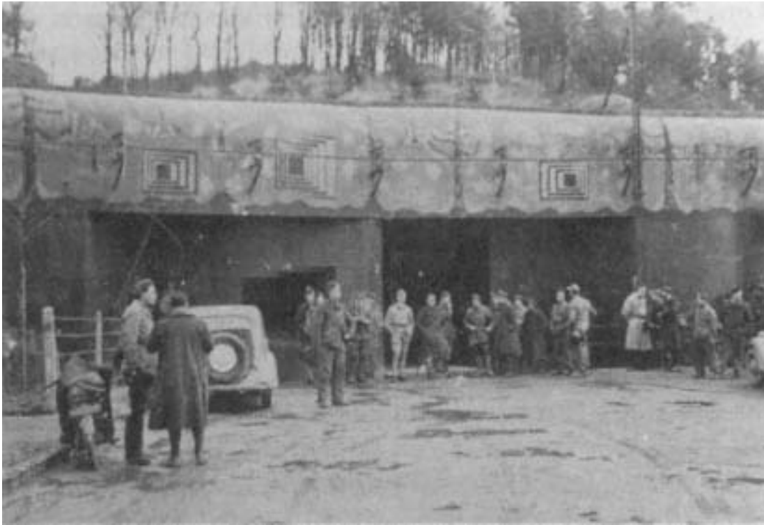
Munitions entrance to a Maginot ouvrage. Note the painted crenels and trees above the entrance.
